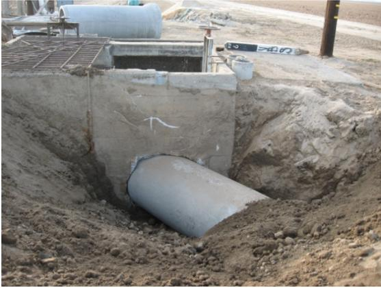
Installation of a crossing on Domingos Ditch at Road 64 on west side of road (replaced old corrugated metal pipe).
