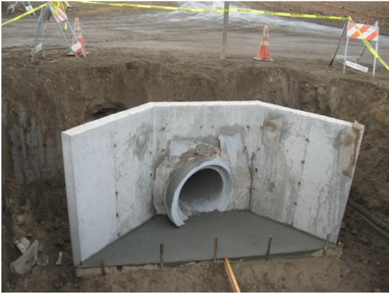
Installation of a crossing on Domingos Ditch at Road 64 on east side of road (replaced old corrugated metal pipe).
