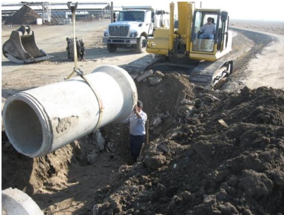
Installation of a crossing on Harris Ditch at Leal's Dairy (replaced old corrugated metal pipe).
