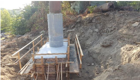
Repair of St Johns siphon vent with concrete box.
