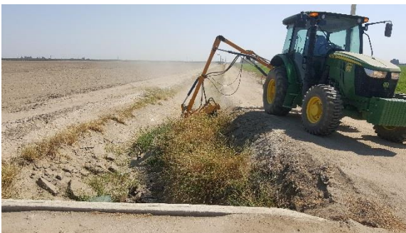
Mowing the canal slopes for grading operations.
