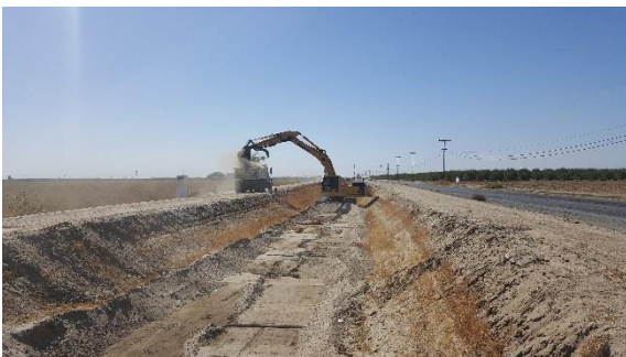
Dreg and hauling of sedimentation in canals and basins.
