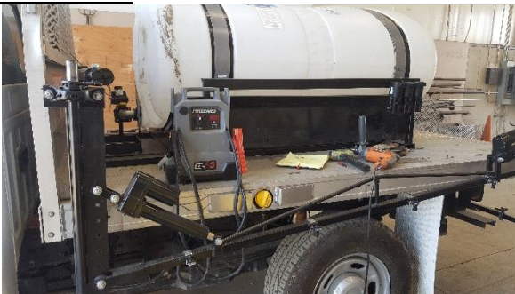
The fabrication of new spray tank for Herbicide Dept.
