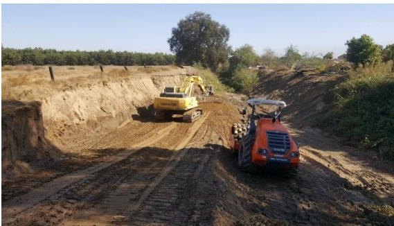
Repairing Crocker Cut bank erosion with district staff and equipment.
