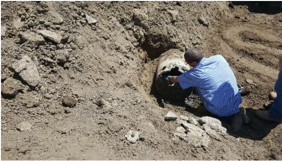
District turnout inspections and repairs.
