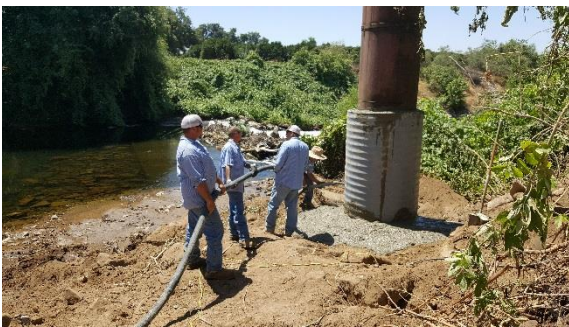
Concrete pumped into sleeve around metal vent at St Johns siphon.
