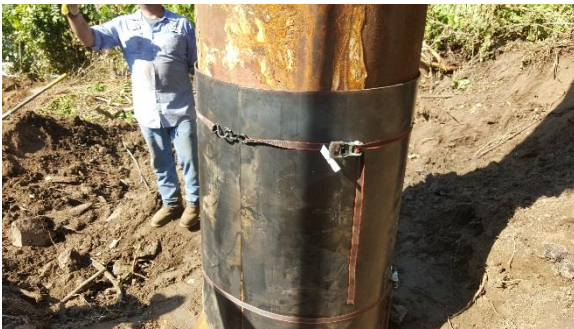
Repair of St Johns siphon vent with 3/6" metal sheets.
