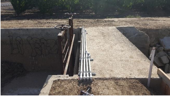
Installation of conduit for automated gates at Packwood creek and Ave 228.
