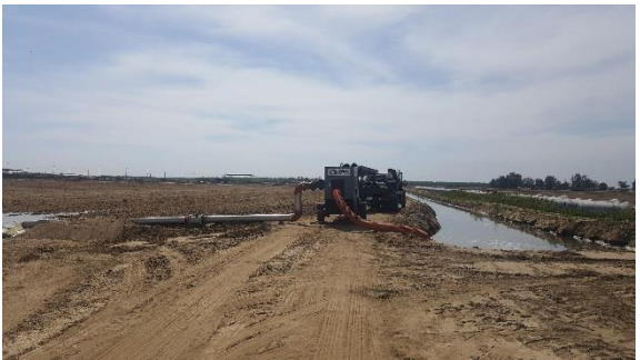
Flooding south end of Cordeniz basin with 8" rental pump. (5 acres)
