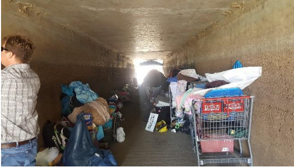
Posting signs for water run in April at Mooney and Northbranch box culvert.
