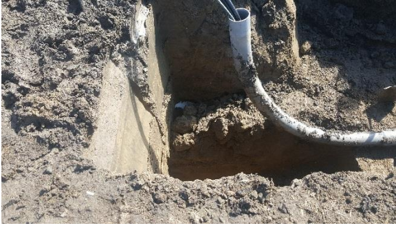
Install Conduit from Modernization Phase II grant project.
