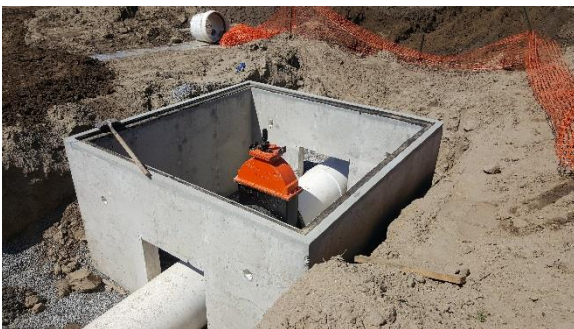
Installation of new Line gates on Serpa East.
