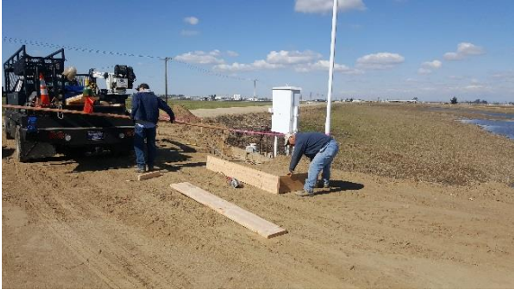
Form work on pad for control boxes.
