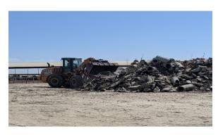
Loading broken pipe from Curti dairy for slope erosion.
