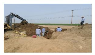
Compacting back turnout replacement on Main Canal west of Road 96.
