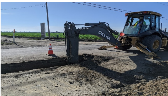
Dig and repair leak at Oakland Colony crossing Road 96.
