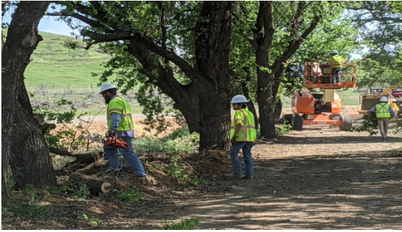
Tree trimming on Main Intake canal along Charter Oak drive.
