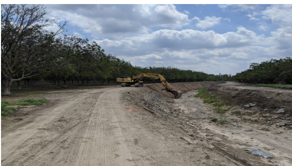
Shape slopes with excavator on Main Intake canal.
