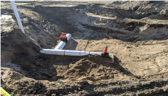
Installing turnouts on the west side of Cordeniz project.
