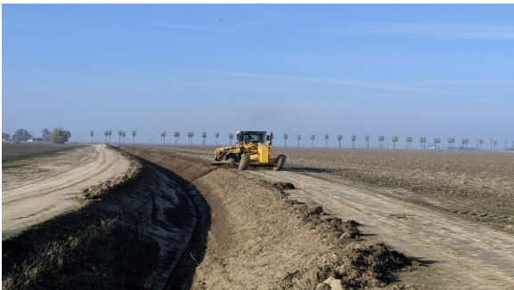
Grading slopes and tops on Lemos Ditch.
