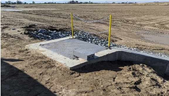
Fabricate and install decking at Cordeniz Basin.
