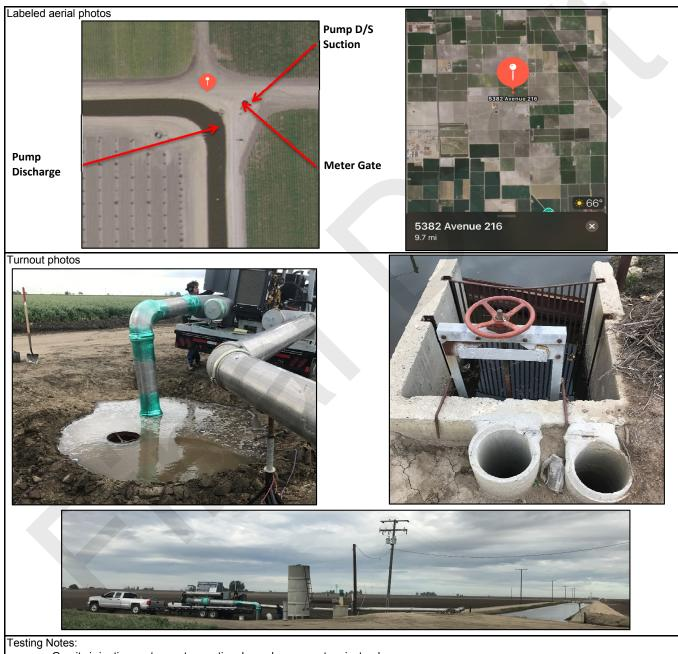
Gravity irrigation system not operational, used pump system instead. Pump can output only one flow rate with one alfalfa valve open
