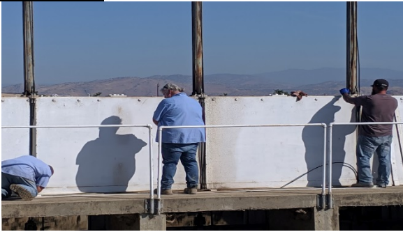
Repairs to hydraulic gates at Wutchumna diversion.
