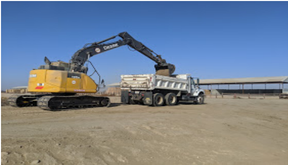
Removal of silt from No. 3 Basin.
