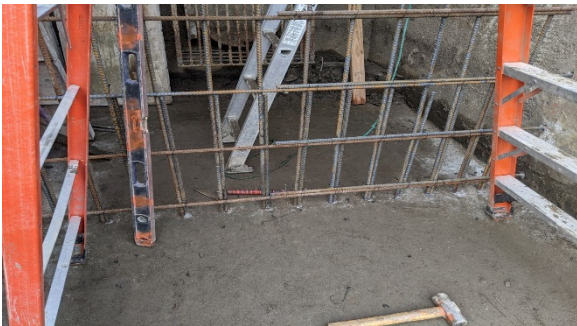
Replacement of wall in Northwest head works at No.3 Basin.
