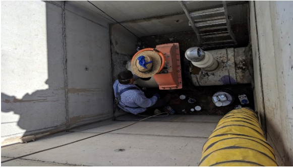
Installing air vents on 24" inlet pipes at Cordeniz Basin
