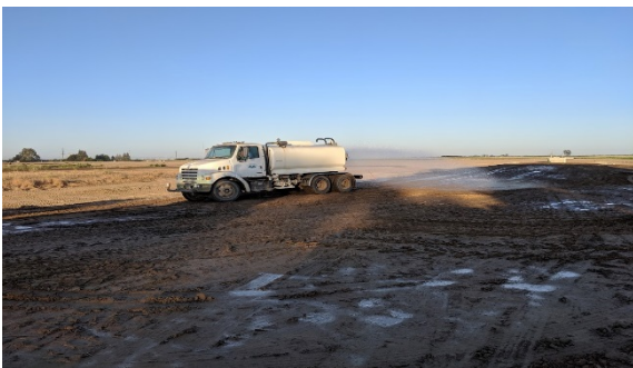
Water truck applying water on banks of Cell No.1 (north).
