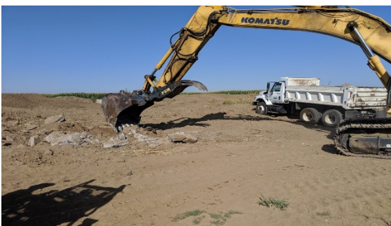
Removing old inlet structure at Cordeniz Basin.
