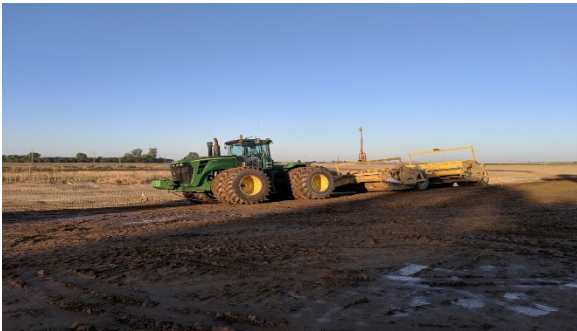
Building banks on Cell No.1 (north) at Cordeniz basin.
