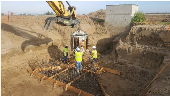
Placement of concrete on bottom of Inlet Structure.
