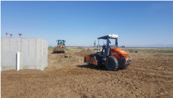
Compacting around distribution box at Cordeniz basin.
