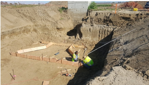
Form installation on bottom of Inlet Structure of Cell No.1 (north).
