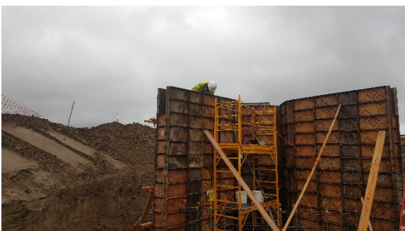
Setting of wall forms for inlet structures.
