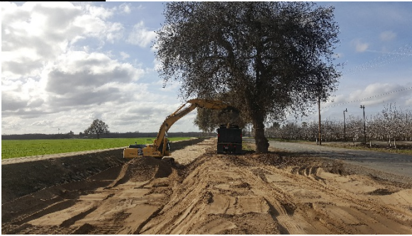
Removing sediment from Cameron Creek along Ave. 264.
