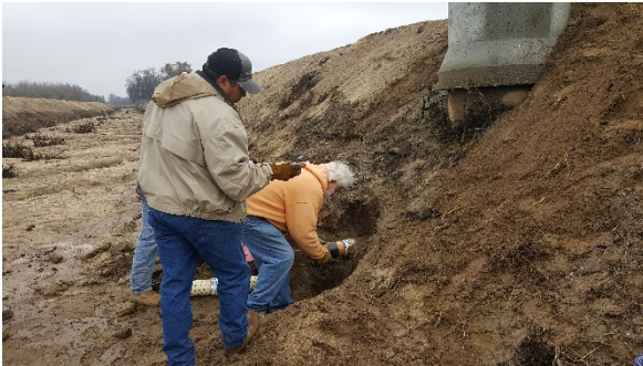
Repairing stilling well at Creamline Basin.
