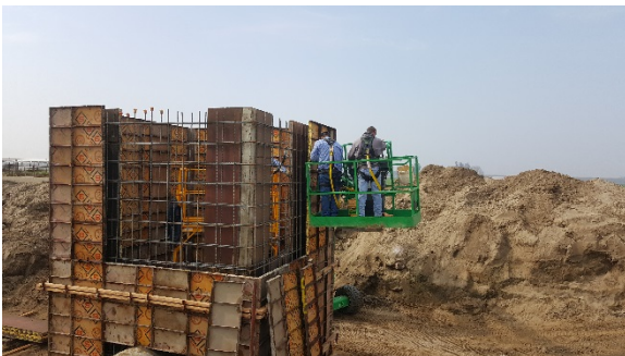
Installation of forms for distribution box.
