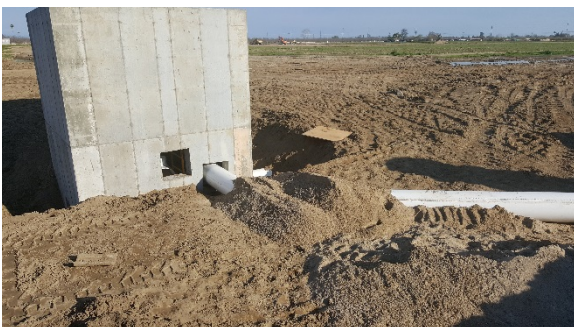
Reconnection of existing Turnouts to the distribution box.
