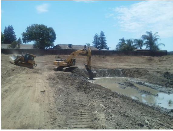
City of Tulare stormwater basin grading operations.
