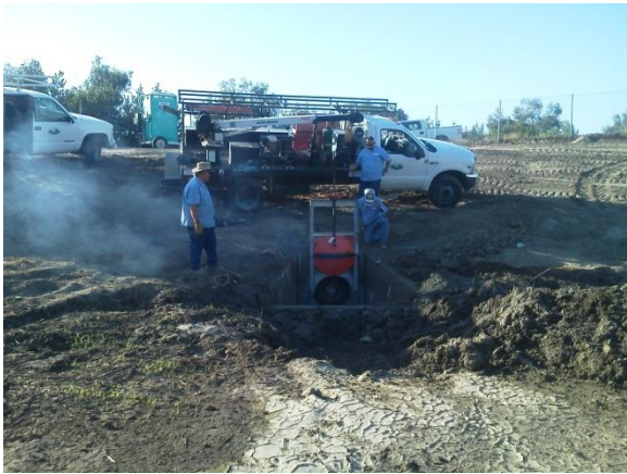
City of Tulare stormwater basin canal gate installation.
