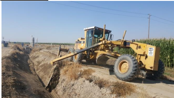
District canal grading operations.
