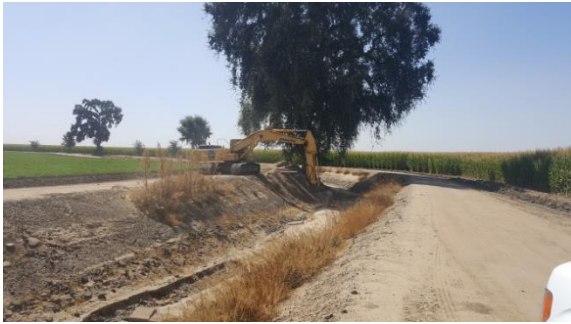
District canal shaping with excavator.
