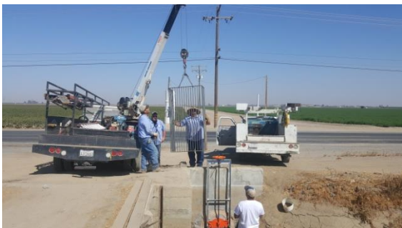
District turnout replacement and repair operations.
