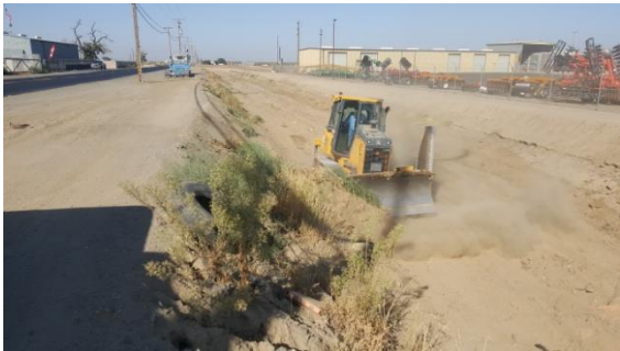
Dozer grading operations in the bottom of District canals.
