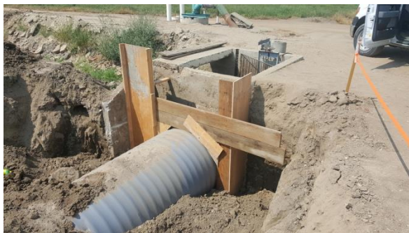
Crossing replacement with HDPE pipe.
