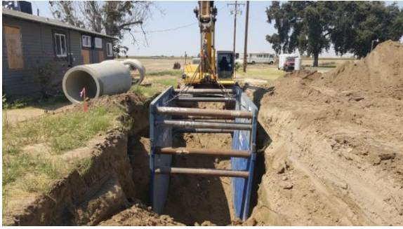
Cordeniz Basin pipeline installation.
