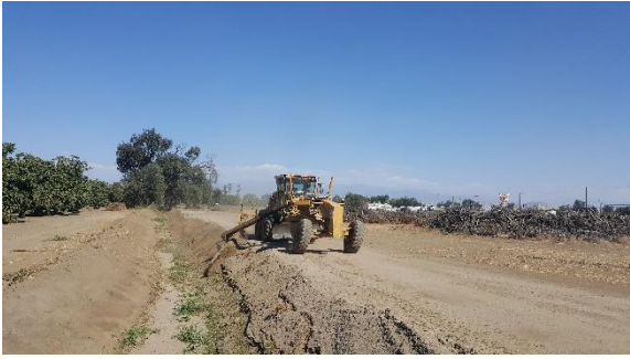
Grading operations on canals
