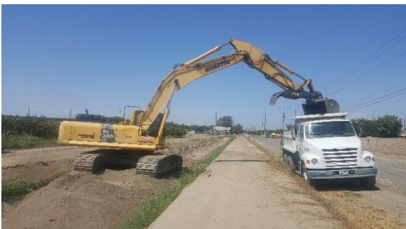
Dredging and hauling of sediment from canals
