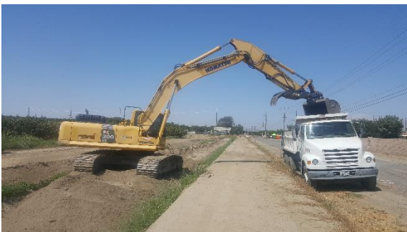
Dredging and hauling of sediment from canals
