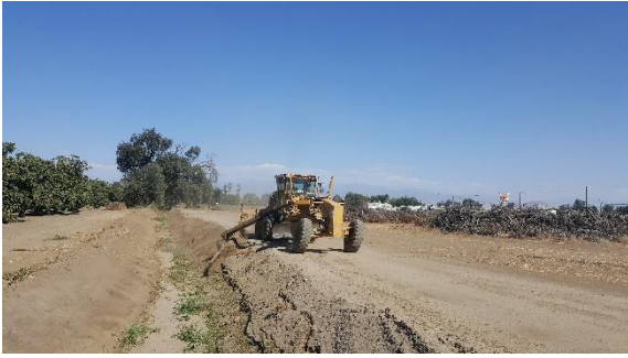
Grading operations on canals
