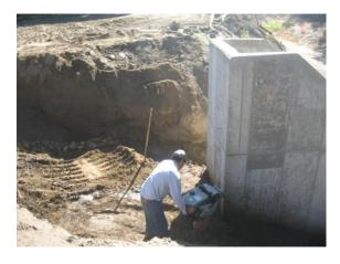
Mooney Grove Basin Turnout installation - backfill and compacting operation.
