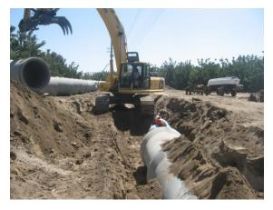
Tristao Pipeline Installation – installation of 42" reinforced concrete pipeline.
