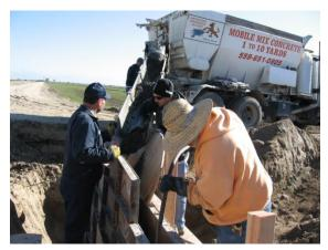
Replacement of corrugated metal pipe on Ravisconi Ditch (west of Road 28).
