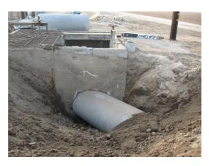
Installation of a crossing on Domingos Ditch at Road 64 on west side of road (replaced old corrugated metal pipe).
