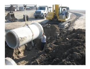
Installation of a crossing on Harris Ditch at Leal's Dairy (replaced old corrugated metal pipe).
