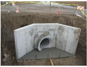
Installation of a crossing on Domingos Ditch at Road 64 on east side of road (replaced old corrugated metal pipe).
