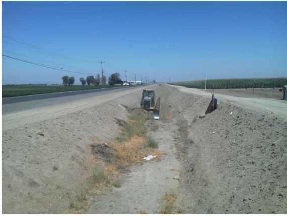
Dozing bottom of canal for weeds
