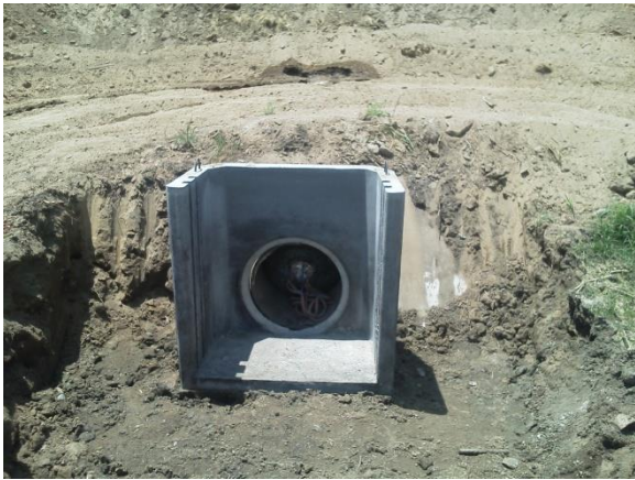
City of Tulare stormwater basin outlet installation.
