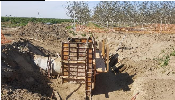
Construction of Serpa Pipeline Headworks.
