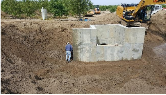
Backfill and compaction for Serpa Pipeline Headworks.
