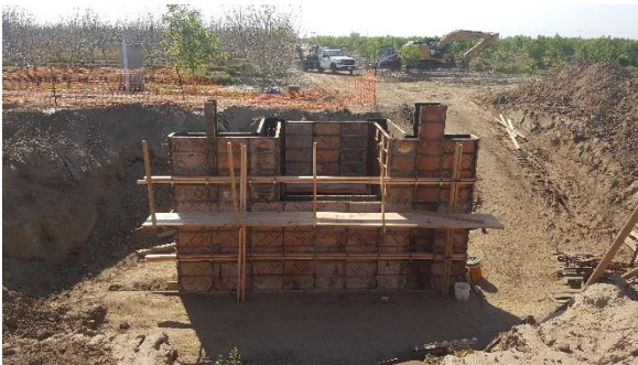
Construction of Serpa Pipeline Headworks.
