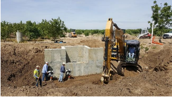
Backfill and compaction for Serpa Pipeline Headworks.
