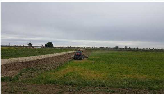
Discing operations at Cordeniz Basin Project.
