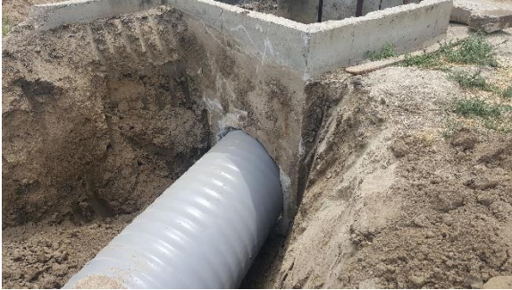
Culvert replacement on Vink Ditch at Road 44.
