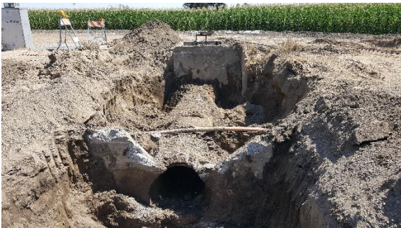
Culvert replacement on V-Line Ditch at Avenue 256.
