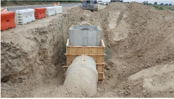
Cordeniz Basin pipeline transition box installation.
