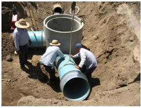
Installation of connection manhole at Area 10 and the new 24" PVC pipeline.
