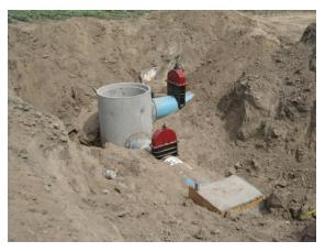
24" PVC pipeline connection to Area 10 Pipeline.
