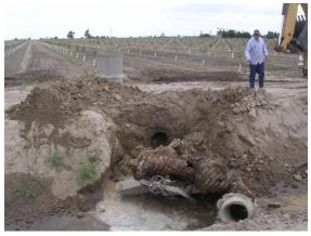
District staff repairing a failed canal turnout at the Bassett Ditch.
