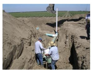
24" PVC pipeline connections to existing turnouts.
