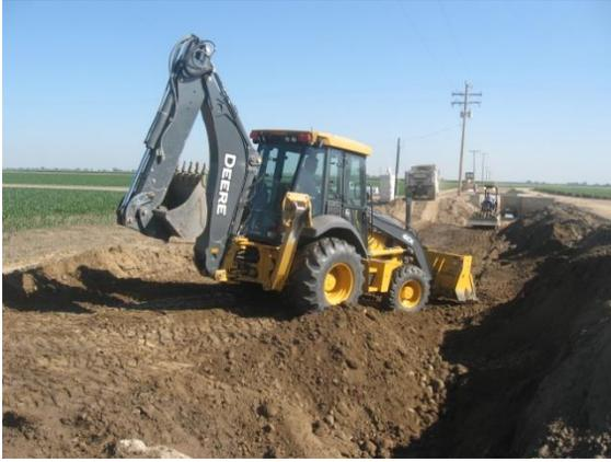
Excavation and compaction of Evans Ditch at Avenue 260. Canal realignment and rehabilitation project.
