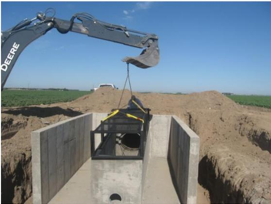
Installation of long-crested weir decking at Cate Ditch.
