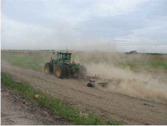
Recharge basin maintenance – basin discing utilizing new John Deere tractor.
