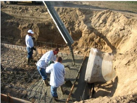
Pouring floor of long-crested weir at Cate Ditch.
