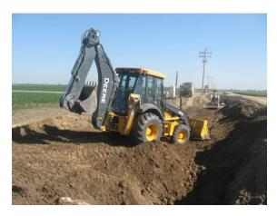
Excavation and compaction of Evans Ditch at Avenue 260. Canal realignment and rehabilitation project.
