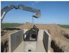
Installation of long-crested weir decking at Cate Ditch.
