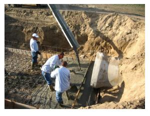
Pouring floor of long-crested weir at Cate Ditch.
