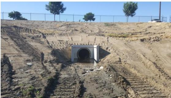
“T” Street Basin inlet structure installation.
