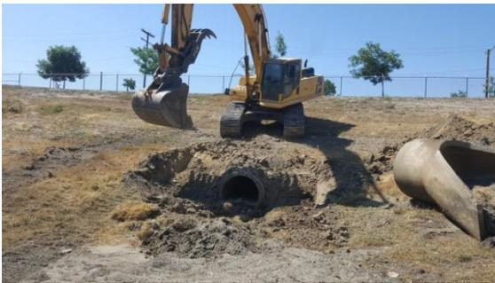
“T” Street Basin inlet structure installation.
