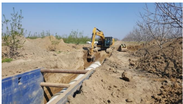
Cordeniz Basin 48” pipeline installation.
