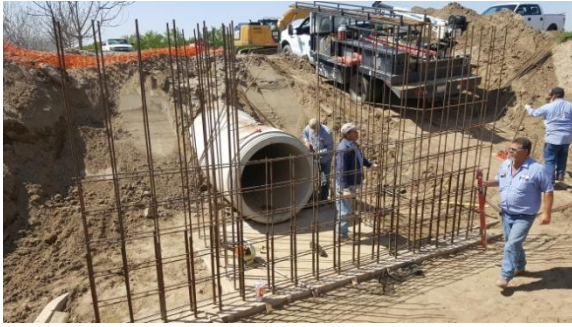
Serpa Ditch headworks installation for Cordeniz Basin project.
