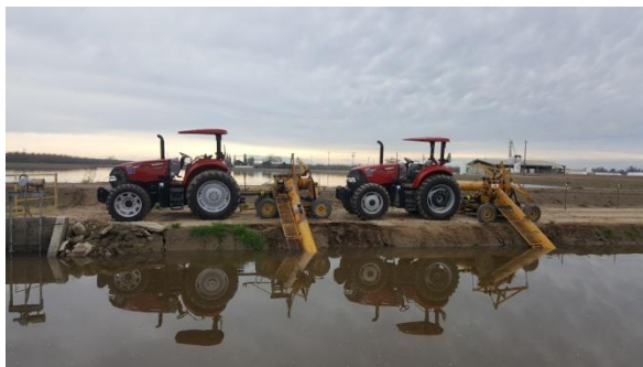
PTO pumps at Swall Basin.
