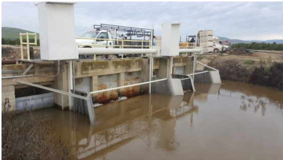
Repairs at Main Intake Canal control gates.
