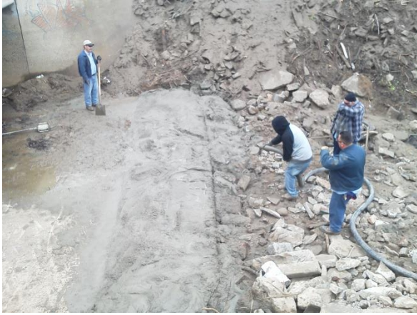
Repair of Northbranch Canal at Tulare County RMA Culvert.
