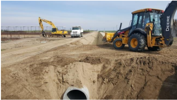
Mattos Canal Crossing Installation.
