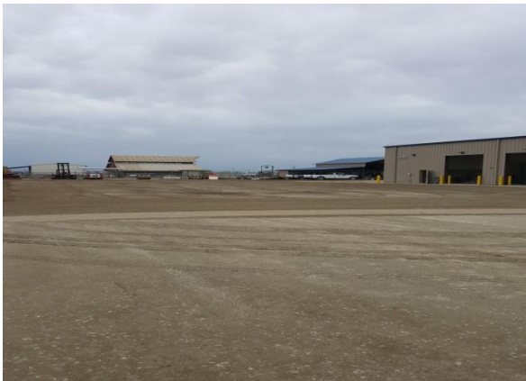
Replacement or aggregate base at shop yard.
