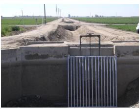
New trash rack installation at Bassett Ditch.
