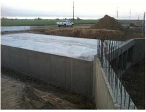
New culvert extension at Northbranch Canal and Road 108. Construction by Teichert Construction and inspected by District (Wayne Fox).
