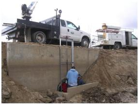
Replacement of canal gate at the headworks of the V-Line Ditch.
