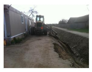
Canal sloping on Sand Ditch at West Street (Road 92). Coordinated with new landowner to regain access to Sand Ditch after 25+ years of restricted access.
