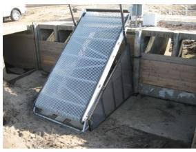
Installation of traveling water screen at Main Canal and Creamline Basin. AquaSystems provided this equipment as a test.
