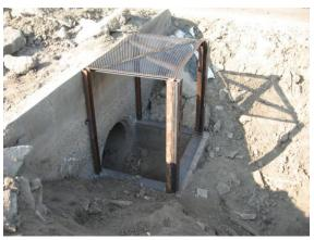
Small long crested weir installation. Fabricated in shop and installed in field this type of small and quick installation allows for better control of canal levels.
