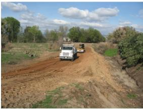
Hauling and compacting embankment at Ketchum Ditch.
