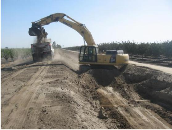
Removal of silt in Packwood Canal at Avenue 228 before reconstruction.
