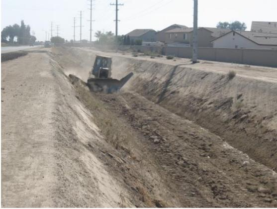
Main Canal shaping operations with rented dozer mounted with sloping blades.
