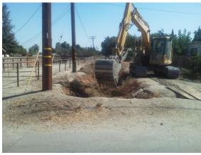
Channel cleaning and maintenance with smaller rental excavator.
