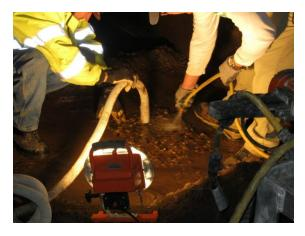
Coring samples being taken at the Kaweah River Main Intake Canal Siphon.
