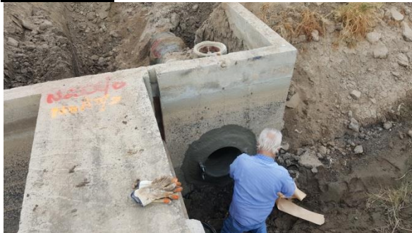
District turnout repair.
