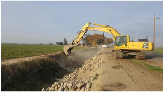
Rip rap placement.
