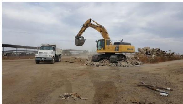
Hauling rip rap to canals and ditches throughout the District.
