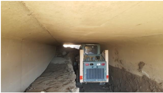
Culvert cleaning operations.
