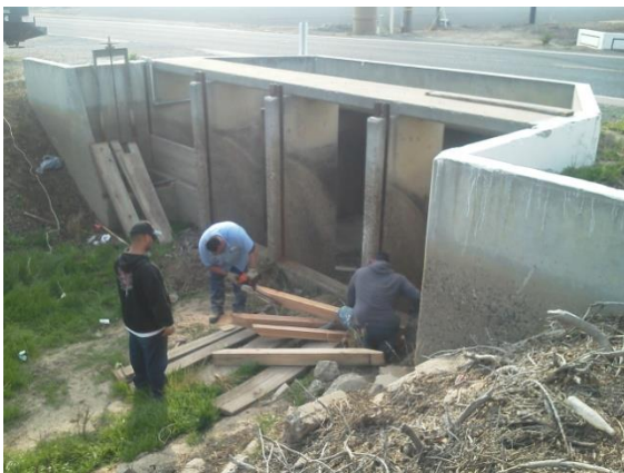
District weir board replacement.
