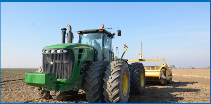
Basin excavation by scraper in tow
