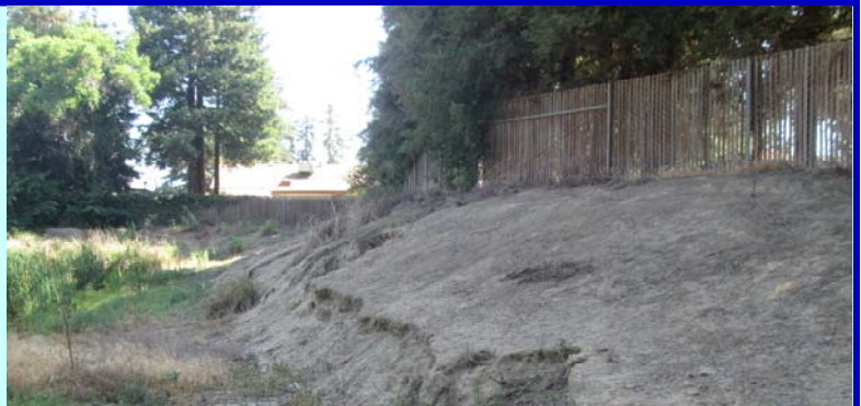
City of Tulare Ponding Basin No. 3
