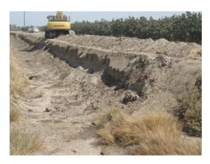
Canal embankment reconstruction on Packwood Creek at the Inlet to 8 Basin.
