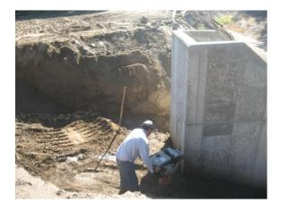
Mooney Grove Basin Turnout installation - backfill and compacting operation.
